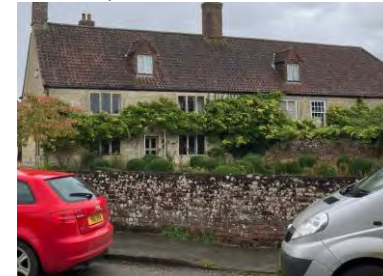
(4) mid-rise brick wall capped with a thin, flat mortar
