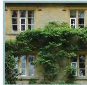
Casement window with chamfered stone mullions.
