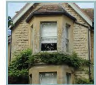
Double storey bay window with glazing set back into the walls to add relief.
